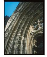
Illustrates loss of detail with weathering. As a philosophical question in relation to authenticity in conservation: 'Should the stone work be replaced with new work, if the old cannot be accurately reconstructed?'
