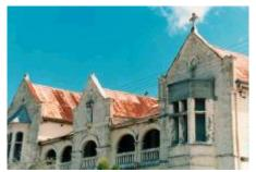
St Brigid's Convent (1898), Northbridge, Perth, Western Australia, in 1997. Gable crucifix details destroyed by corroding metal fixing rods, gutter and rain goods not maintained - allowing water ingress, roof sheeting corroded - requiring reconstruction, and inappropriate cement rendered repair work.
